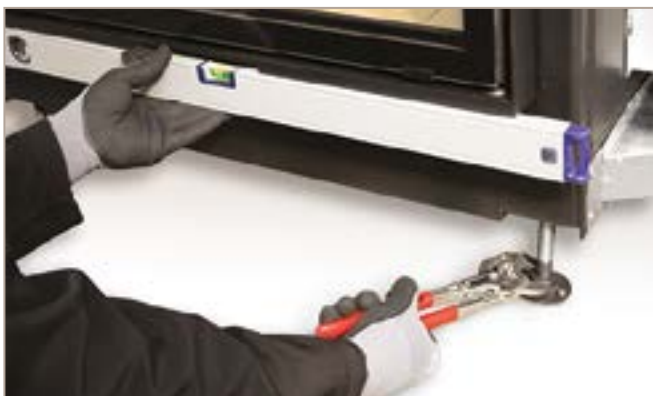
Fig. 13: Levelling the fireplace insert
