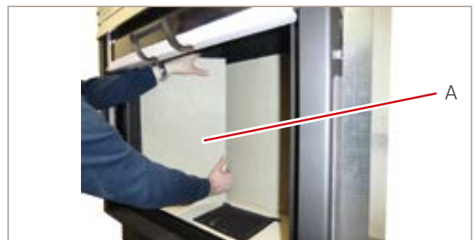
Fig. 22: Removing the fire box inner lining
