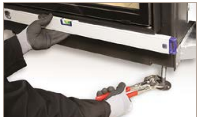
Fig. 16: Levelling the fireplace insert
