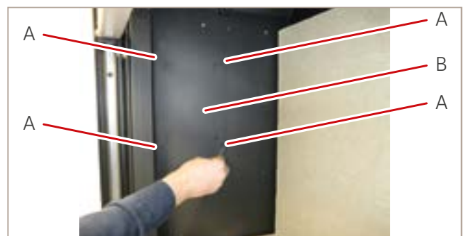
Fig. 25: Dismantling the revision cover
