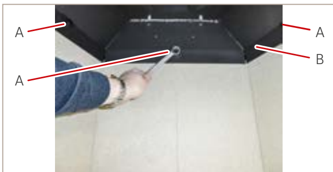
Fig. 19: Loosening the fixing screws
