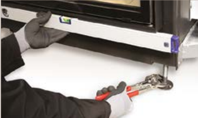
Fig. 12: Levelling the fireplace insert
