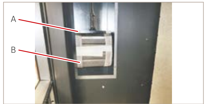
Fig. 24: Primary and balancing weight
